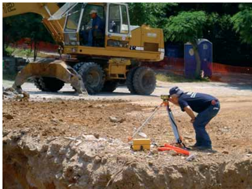
At work on the new Classroom Annex
